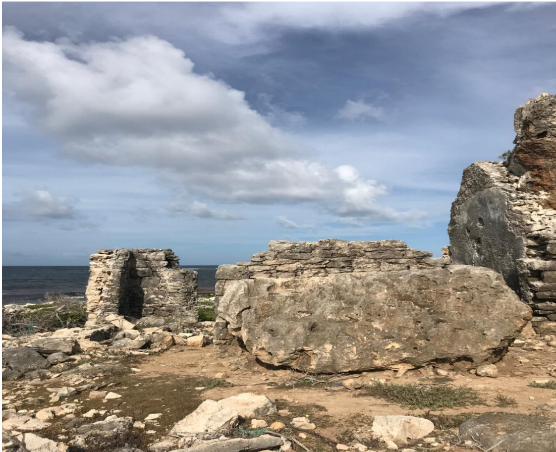
Photo 2. Gunshop Cliff, Barbuda. Walls collapsed after Hurricane Irma. (Photo by Sophia Perdikaris).
